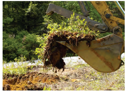
Photograph 5 & 6. June 6, 2016—Drought Rating “D0”—Abnormally Dry. Translocating blocks of soil/vegetation at upland buffer edge of the traditionally constructed wetland replication area (Traditional Replication Wetland). These photos show the translocation technique, but are showing soil and shrubs that are being salvaged and translocated from upland excavated to construct the Traditional Replication Wetland. They are being planted in upland buffer to the Traditional Replication Wetland. Photo source: Gillian Davies.
