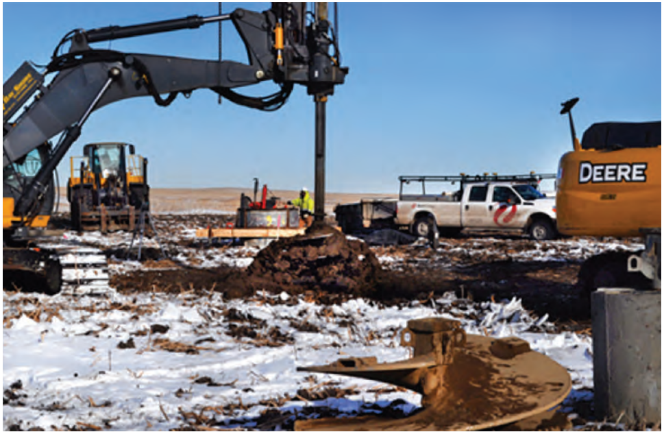
Figure 7. Drilling Structure Foundation
