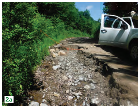
Figure 2a and 2b. Erosion of roads due to poor water management
