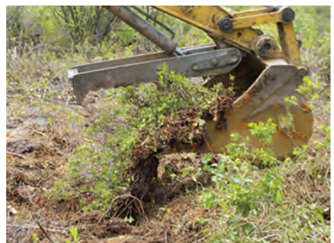
Photograph 7 & 8. June 6, 2016—Drought Rating “D0”—Translocating blocks of soil/vegetation at upland buffer edge of the traditionally constructed wetland replication area (Traditional Replication Wetland). These photos show the translocation technique, but are showing soil and shrubs that are being salvaged and translocated from upland excavated to construct the Traditional Replication Wetland. They are being planted in upland buffer to the Traditional Replication Wetland. Photo source: Gillian Davies.
