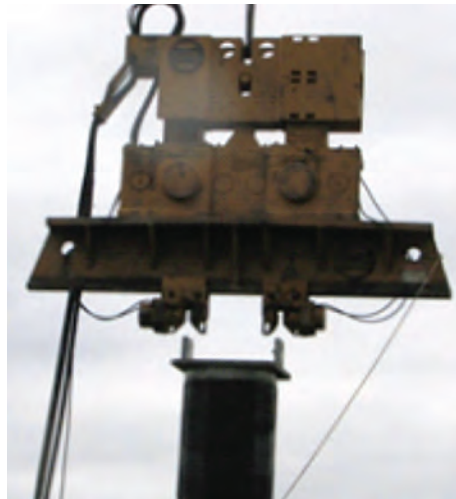
Exhibit 7. Placing Vibratory Hammer to Drive Steel Caisson
