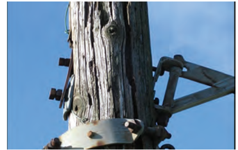
Exhibit 3. Pole Deterioration
