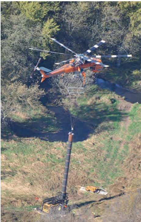
Exhibit 6. Transporting Steel Caisson and Equipment to Structure Locations
