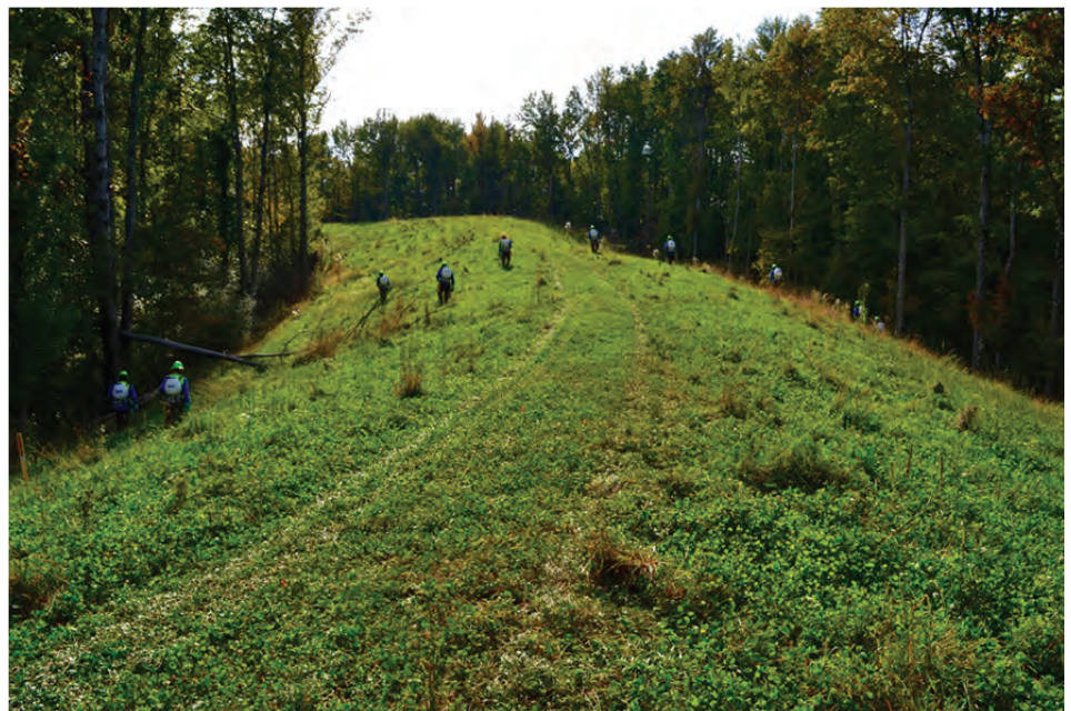
Figure 1. Treatments 1 and 3 plots controlled incompatible invasive species and woody encroachment via backpack sprayer foliar application of selective herbicides—September 2016, Ohio.
