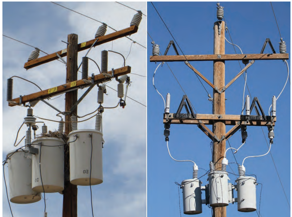
Figure 6. Incorrectly retrofitted power pole. Lower jumpers are covered, but no other retrofitting exists on the pole. The nestling just visible in the Red-tailed Hawk ( Buteo jamaicensis ) nest on the center transformer is at high risk of electrocution (left). Thoroughly retrofitted power pole. Triangles on each crossarm illustrate redirection, 10-ft upper crossarm illustrates separation, and covers on jumpers, cutouts, arresters, and transformer bushings illustrate insulation (right).
