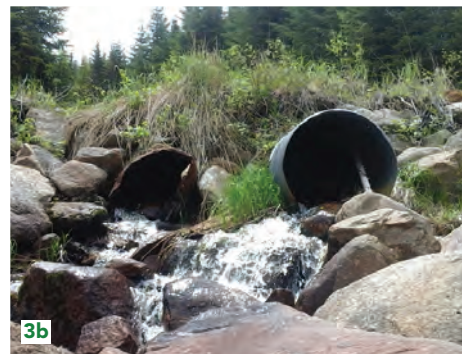
Figure 3a and 3b. Percentage of stream-crossings maintained on public land (Paradis Lacombe and Jutras 2016) and (b) new culvert installed next to old culvert in bad condition
