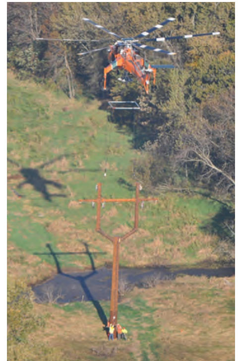
Exhibit 8. Attaching Steel Y-Frame Structure to Caisson
