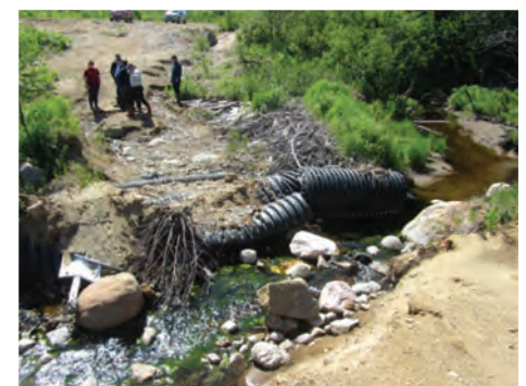
Figure 6. Improved Ford on Low-Volume Road, Côte-Nord, Québec
