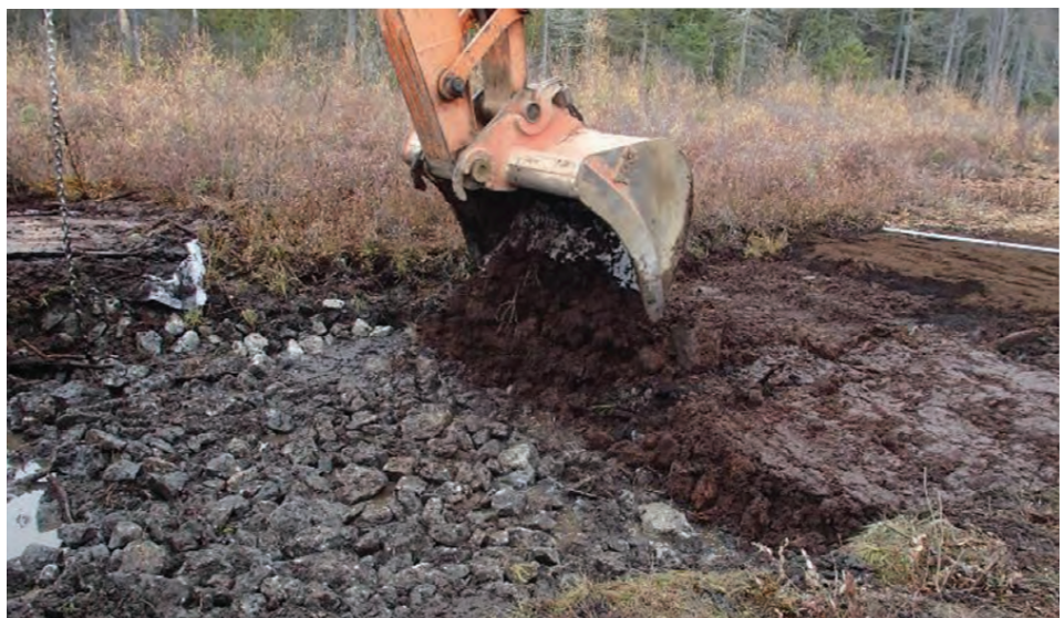
Figure 2c. Covering the mineral material with the stockpiled peat (at least 40 cm)
