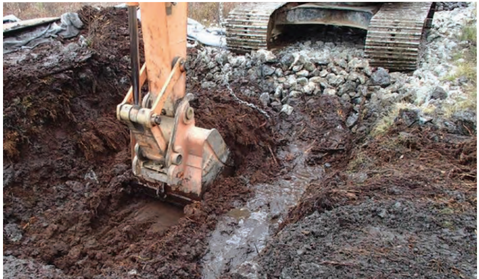
Figure 2a. Excavation and stockpiling of the underlying peat
