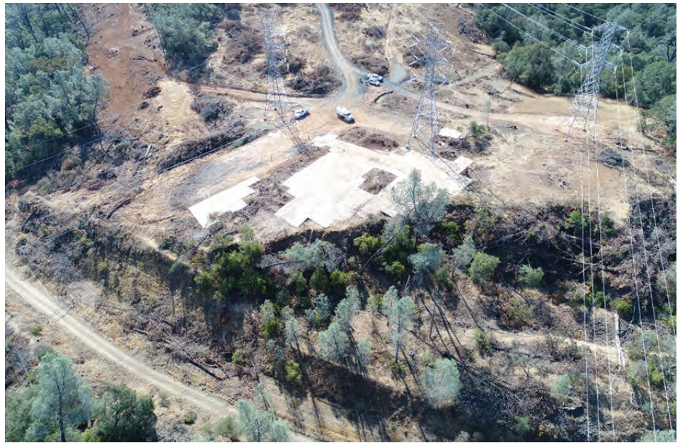
Photograph 2. Use of Mats to Distribute the Weight of Equipment in Areas with Potential Sensitive Surface or Subsurface Resources. Photo credit: DWR.
