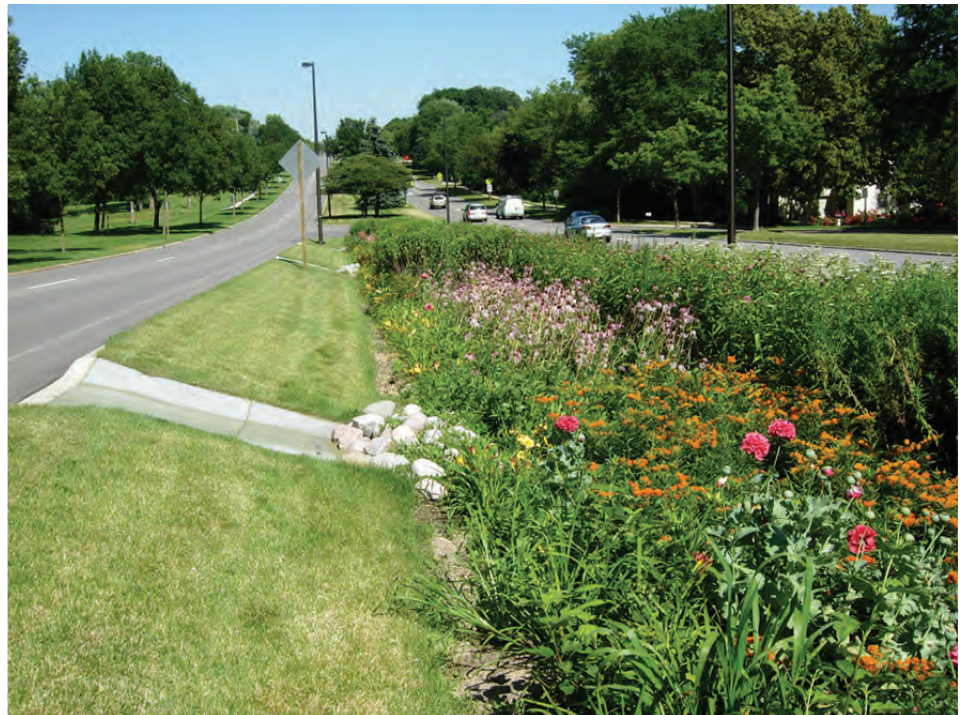
Figure 1. New and existing infrastructure should include considerations for environmental remediation. This recently built median diverts storm water to a bioswale that recharges groundwater, provides pollinator habitat, and meets the needs of the roadways.
