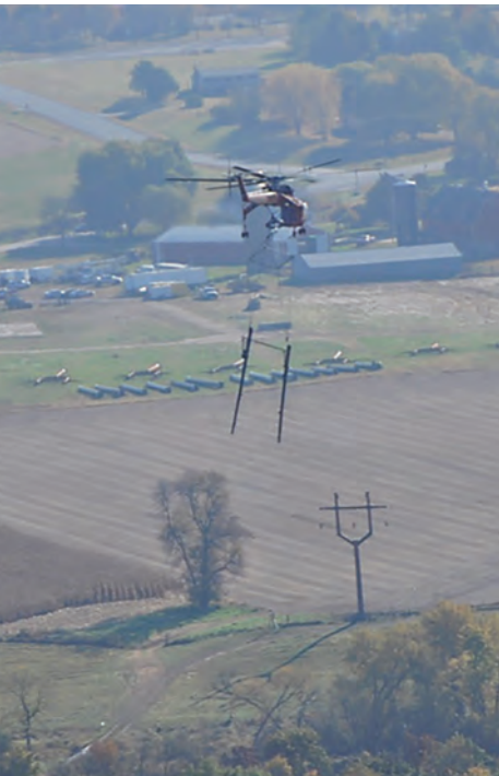
Exhibit 5. Removing Existing H-Frame Structure
