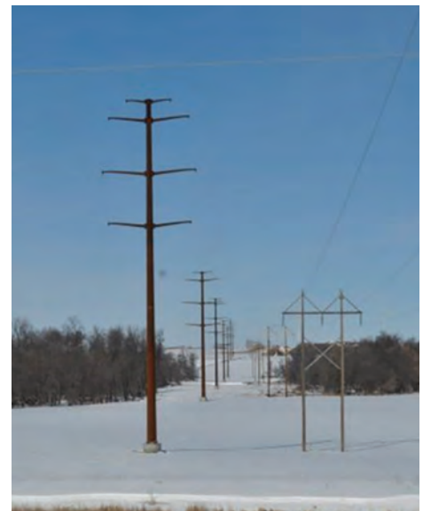
Figure 9. New 230/115-kV double circuit line (left) prior to removal of existing 115-kV transmission line (right)
