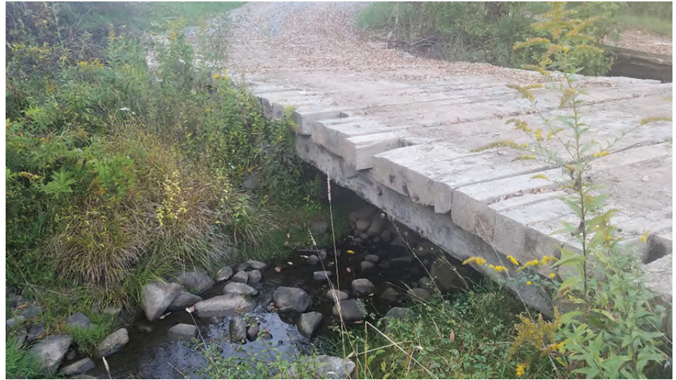
Figure 1. Matting: installation of construction matting over stream resources can be an effective way to minimize impacts
