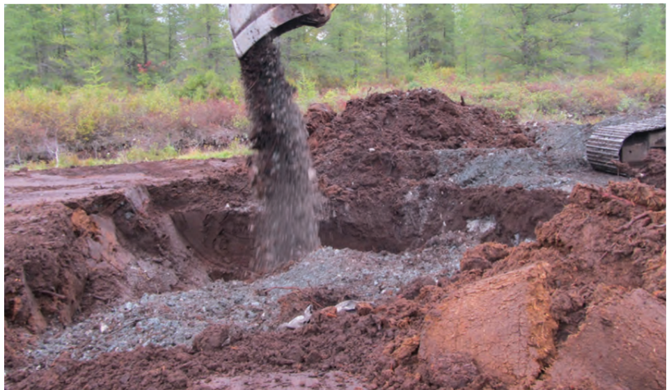
Figure 2b. Fill of the excavation with the mineral material
