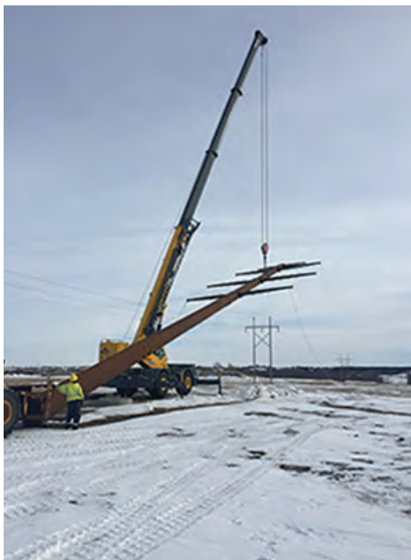
Figure 8. Placing Single Pole Steel Structure
