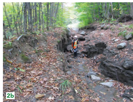
Figure 2a and 2b. Erosion of roads due to poor water management
