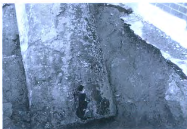
Fig. 2. A leaking underground storage tank being removed from the ground.
