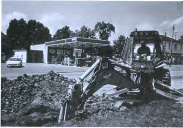
Fig. 6. Test pitting at Bond Head with the gas station in the background.
