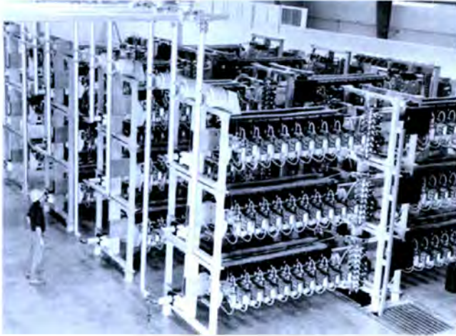
Fig. 3. UPFC installation.
