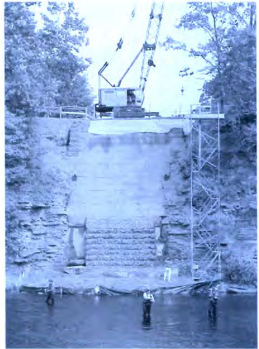
Fig. 4. Hard armor system used on Pipeline 33 crossing Salmon River. To retain toe subject to 18-foot stage increase and ice/debris erosion in floods when currents are directed into this bank, repairs integrate boulders, concrete, gabions and a soil mesh system along with up-slope site grading. Southern aspect requires porous media to cope with freeze-thaw of ground and surface water infiltration.
