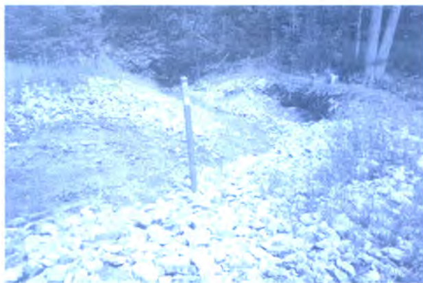
Fig. 10. Tully Farms Road stream intersected the broken shale of the original trench cover, and began to follow the pipe. The stream was redirected, stepped gabions installed, but the radius of curvature for the bend below the gabions was too tight. Longitudinal forces scoured the riprap on the outside curve that was premature, demonstrating that meanders tend to migrate downstream. Water flowing over an obstruction leaves the obstructing surface flowing at right angles to it.
