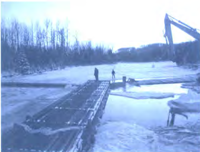
Fig. 3. Aquadams TM (centre of photo) diverting flow of the Little Smoky River into the 30 m long superflume. Crossing successfully installed by Marine Pipeline Construction.
