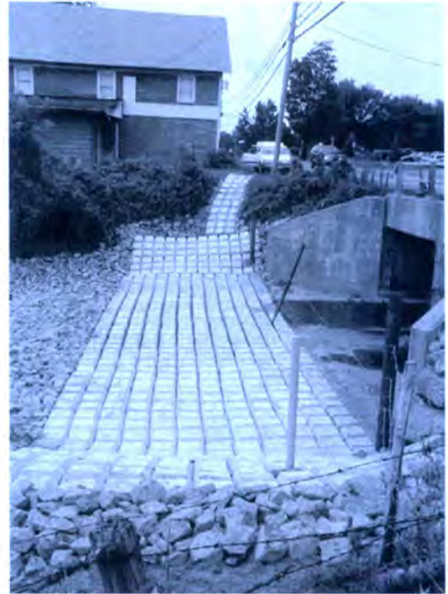
Fig. 5. Concrete mat used to stabilize the bankside drainage ditch from the highway and also the bed of the stream at Budlong Creek in Utica, NY.
