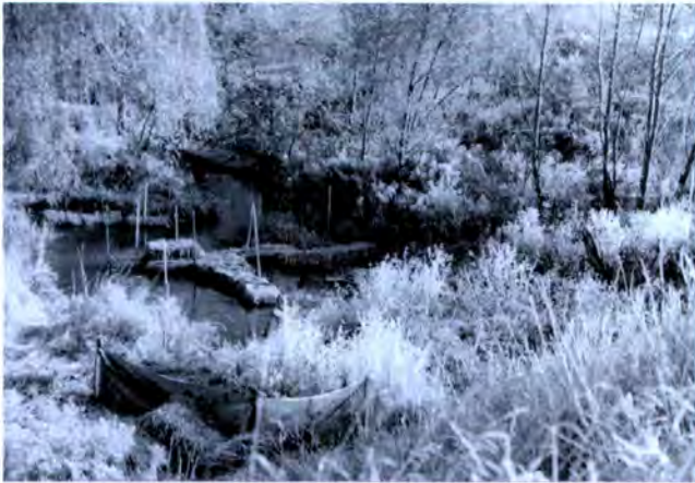
Fig. 5. Instream containment of bentonite fracout.
