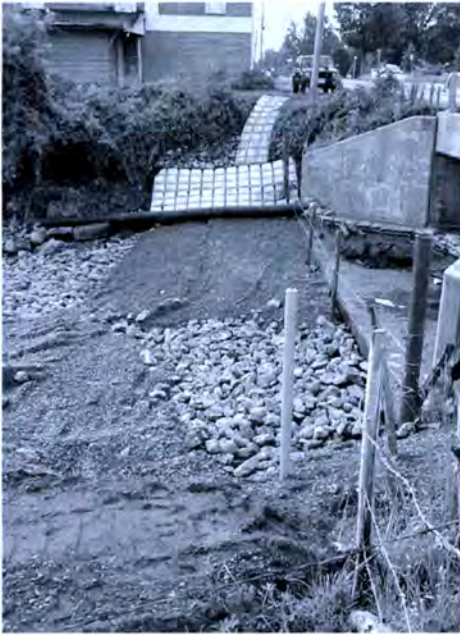
Fig. 6. Yellow rock shield mesh and sand bedding beneath graded crushed stone, then fabric lined concrete block mats, with anchors. Subsequent runoff vibrated the blocks, shredded the stainless steel cable, and debris carried dislodged several blocks from the mat. Settlement and loss of bedding material by undercurrents is accelerating deterioration. Note the temporary diversion pipe.
