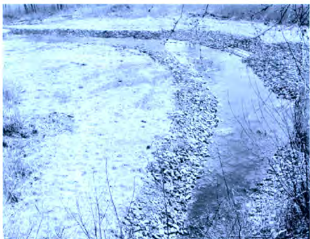
Fig. 9. Pipeline E-30 and tower leg exposures resulted from a narrow gully, which made tight turns, to intermittently divert its storm discharge along the disturbed earth of the pipeline backfill in a wetland. Hydraulic radius and capacity was increased, sinuosity redefined, and banks at turns armored with stone and mats. Allowances were made to let the stream go out-of-bank in floods.
