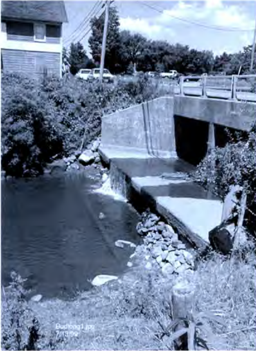
Fig. 3. Nickpoint is a box culvert. Highway culverts are nominally sized for the 25-year discharge event. Sediment is trapped upstream and the outfall erodes as the undernourished stream seeks a new sediment load. Banks then collapse as the bed incises and headcuts. Pipe cover below culvert failed from turbulence, cattle traffic, and inadequate armor to match storm events.
