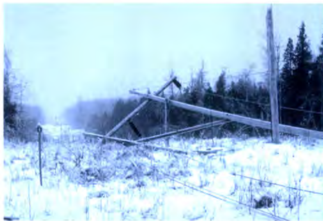
Fig. 2. Collapsed 120 kV powerline in January 1998.
