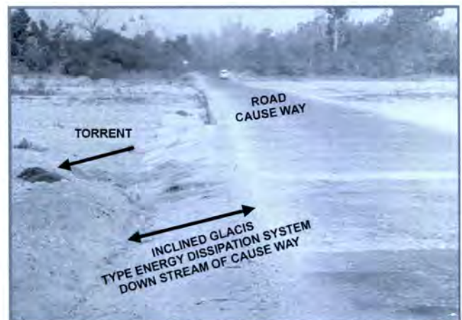
Fig. 6. Sloping glacis type energy dissipation system at downstream end of road causeway on Haridwar–Bijnore highway.
