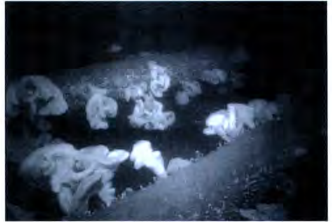
Fig. 2. Sponges and calcareous tube worms colonizing sections of two small marine pipelines, nine years after construction.
