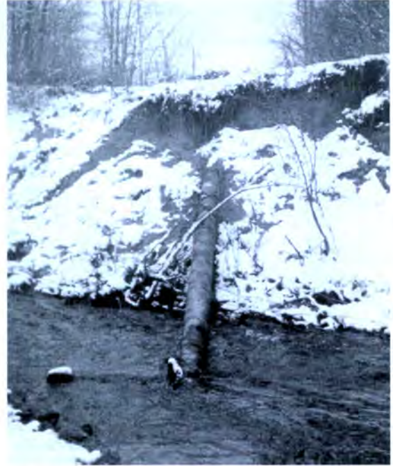
Fig. 8. Deer Creek exposure from meander migration into south bank, compounded by upstream debris/shoaling that diverted currents. Hydraulic capacity increased by widening channel, debris cleared upstream and down, trees removed that would capture flotsam, and gabions installed to move south bank back over the pipe.
