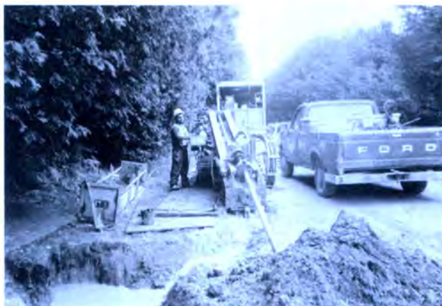
Fig. 4. Roadside directional drill showing sump pit for drill mud.
