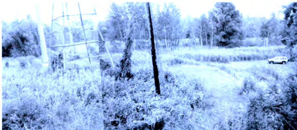
Fig. 11. Pipeline E-30 and tower leg exposures resulted from a gully intermittently diverting its storm discharge along the disturbed earth of the pipeline backfill in a wetland. Hydraulic capacity was increased, sinuosity redefined, and banks at turns armored with stone and mats.
