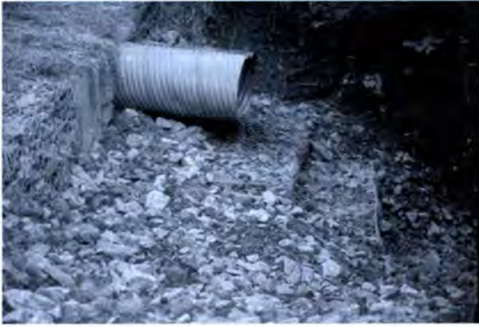
Fig. 7. Porous outfall protection (stepped gabions) absorb and dissipate energy that is undercutting an interceptor culvert that diverts water from the pipeline running directly upslope. The original installation left a 6-foot free fall that scoured and undermined the headwall placed to hold the drain pipe.
