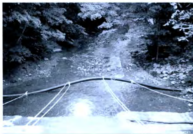
Fig. 1. Washout of 8" gas line in Willow Creek following a July 4, 1999 thunderstorm. Although bedded and buried well, the disturbed trench in bed of the stream was unconsolidated in relation to the naturally packed hardpan of the streambed, and cover was scoured. A concrete cap was installed to make the repair.
