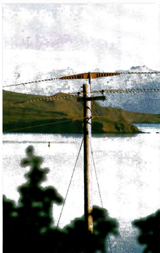
Fig. 2. Pole raptor protected with a conductor guard.
