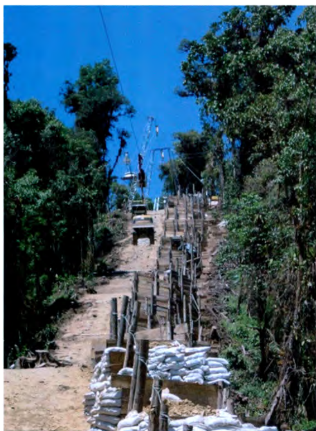
Fig. 5. Equipment transportation using cable system.
