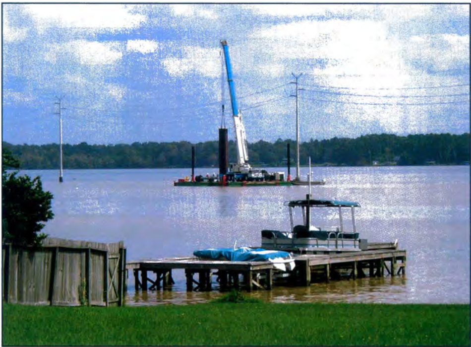
Fig. 9. Installation of the foundation casings for the construction of the steel pole line across Lake Houston. Note the diameter of the casing suspended from the crane compared to the concrete pole foundations installed in 1997. Photo taken October 13, 2003.
